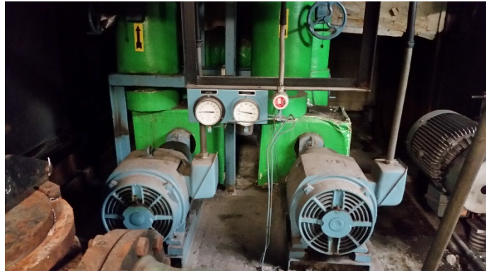
Figure 3: Pumps P-11 and P-12 serve CH-2
