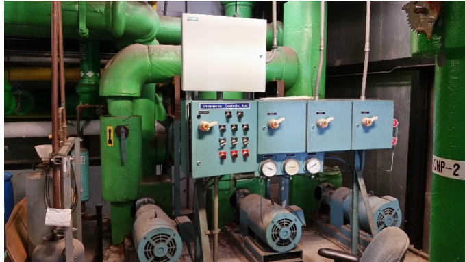
Figure 3: Pumps P-13, P-14 and P-15
